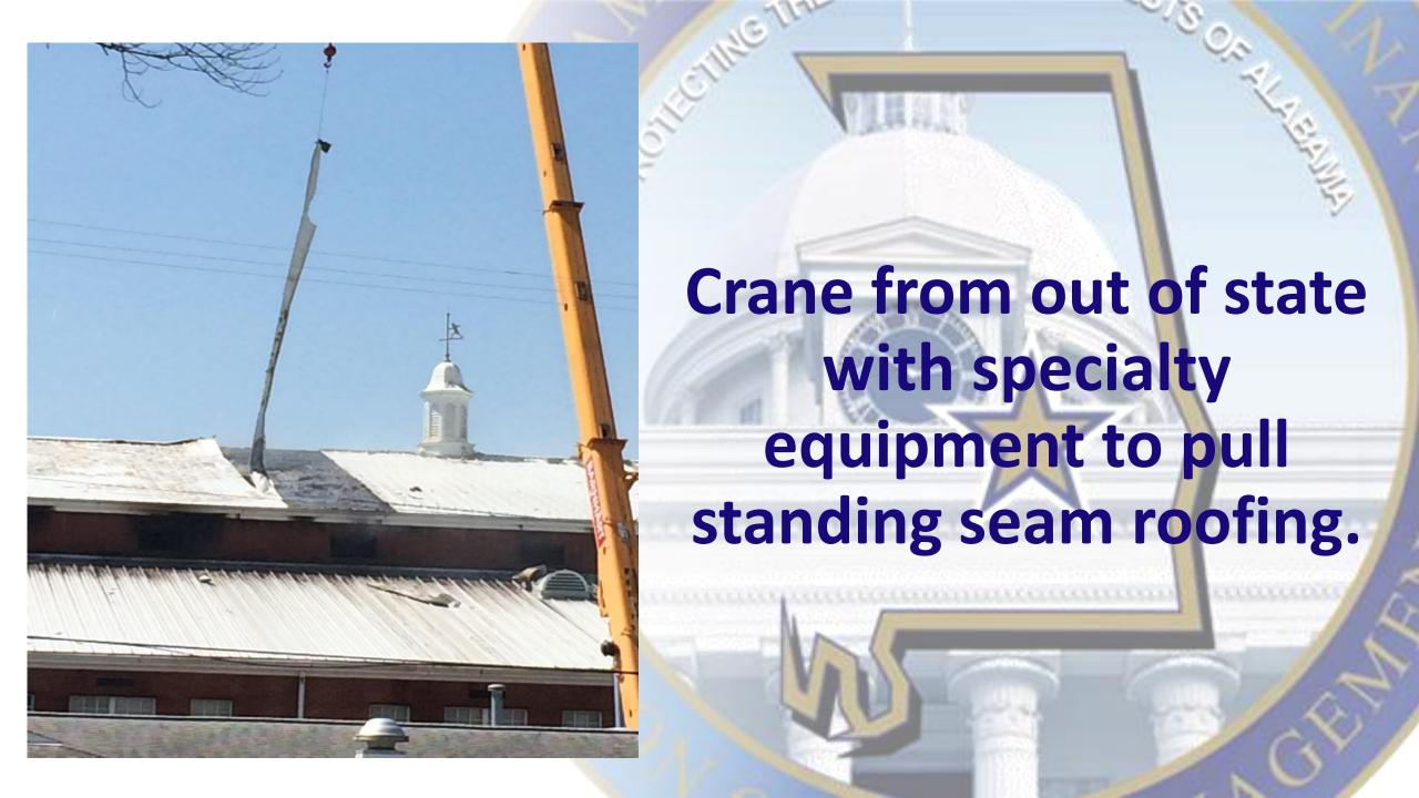
**Roofing materials** layers sandwiched under standing seam roofing were ignited. The metal roof had to be removed to extinguish the fire.
